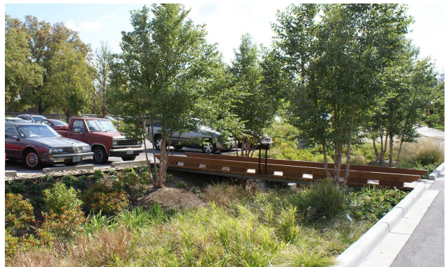
Bioswale at Parking lot
