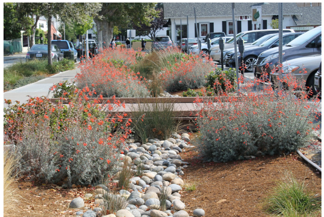
Planting at Swale Zone
