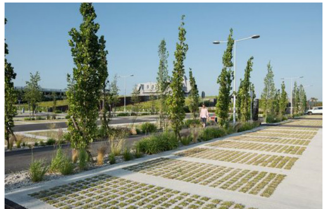
Porous Paving at Parking Lot
