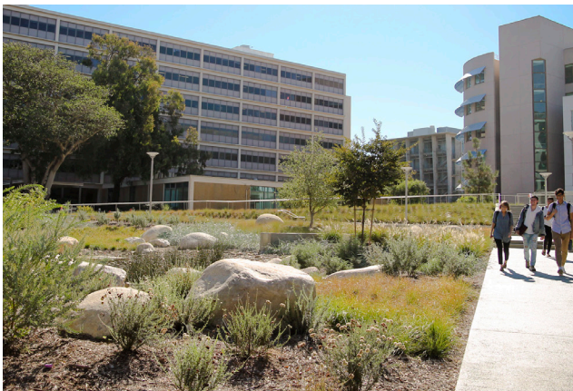
Swale Adjacent to Walkway
