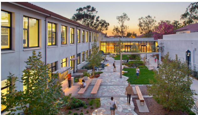
Courtyard between Buildings
