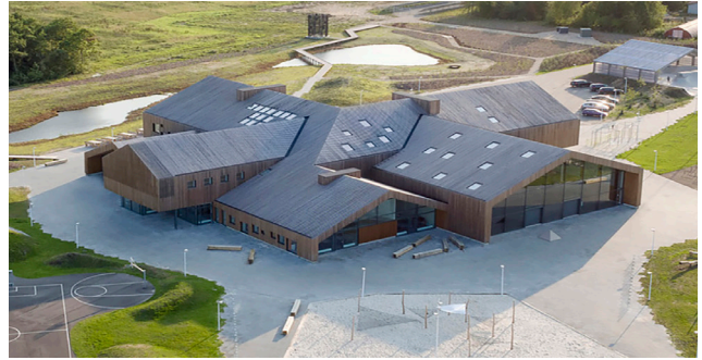
Use of roof overhang and placement of entry plaza/ shaded spaces towards the north to limit direct sun exposure.
