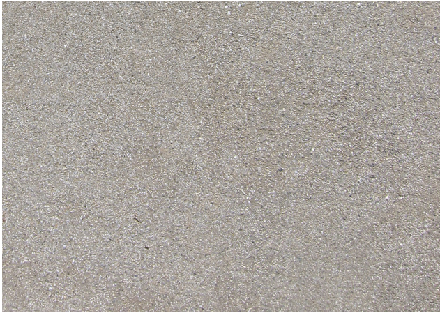
CIP Concrete Paving with Sand Finish
