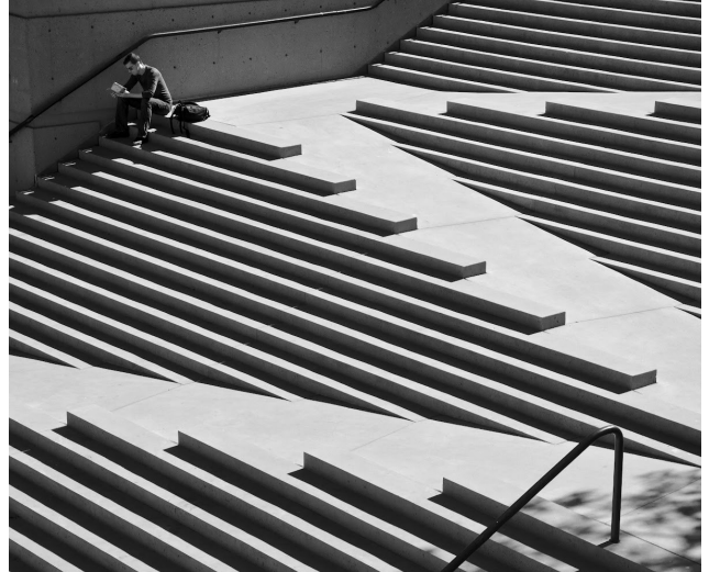
Universal design that combines ramp and stair elements can also contribute to unique placemaking and gathering spaces.
