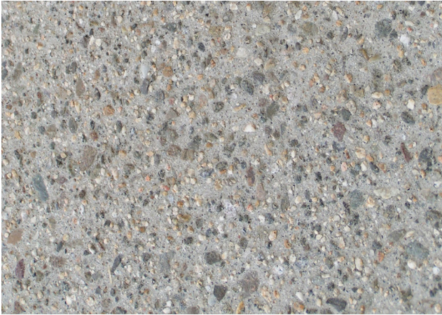
CIP Concrete Paving with Exposed Aggregate Finish
