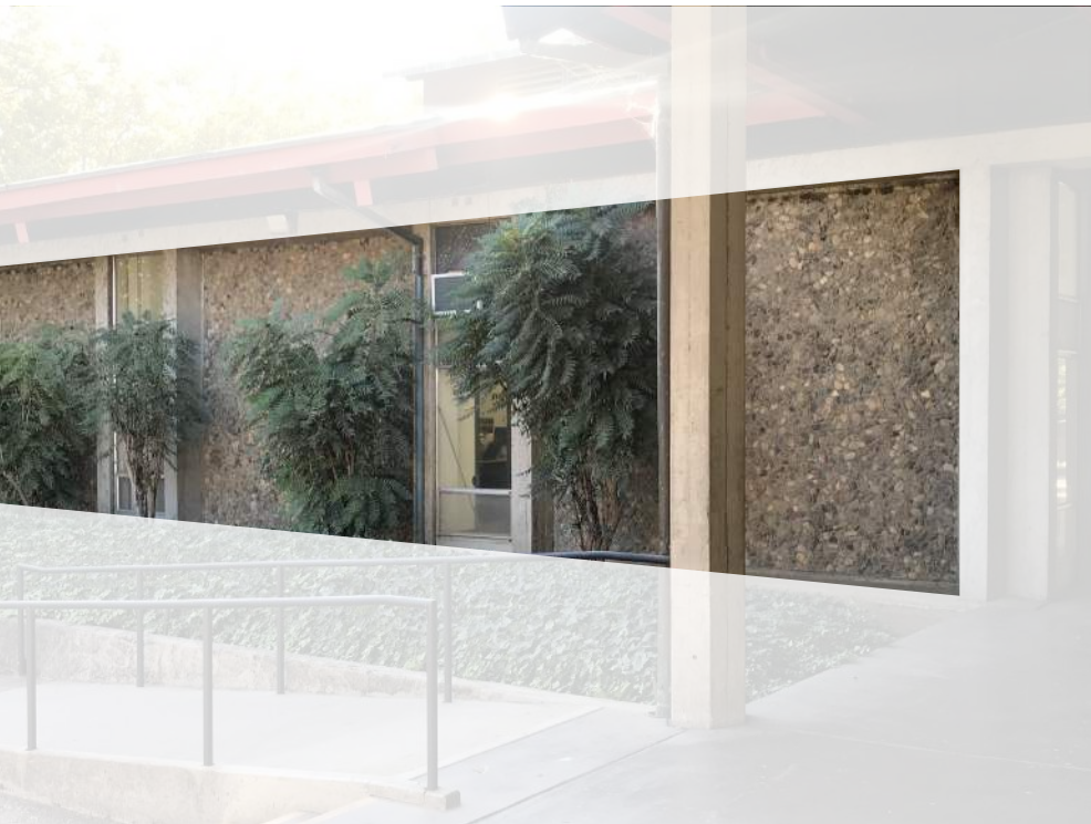
Tilt-up Concrete w/ Exposed Aggregate
