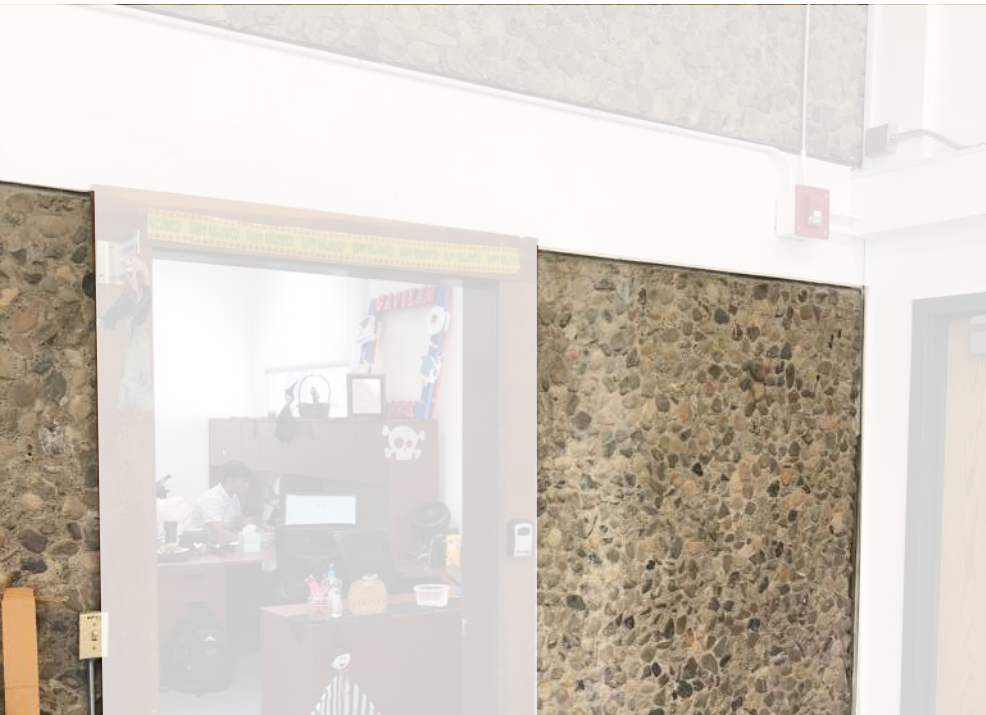
Tilt-up Concrete w/ Exposed Aggregate
